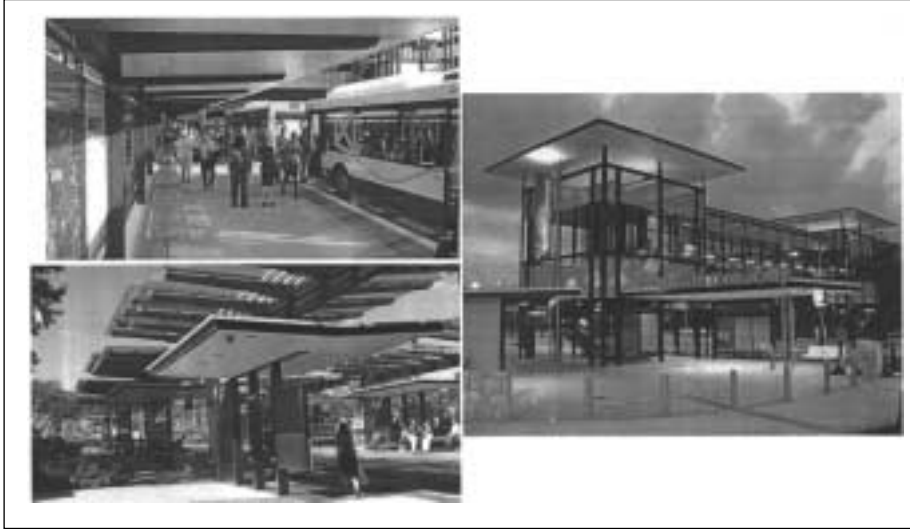
Figure 13. BRT stations Brisbane: South East Busway
