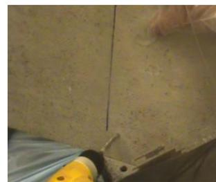
**Figure 1. Transite Being Drilled**
