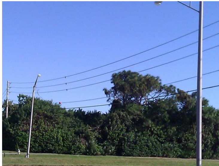
Figure 1: A cable hanging between to power poles.
