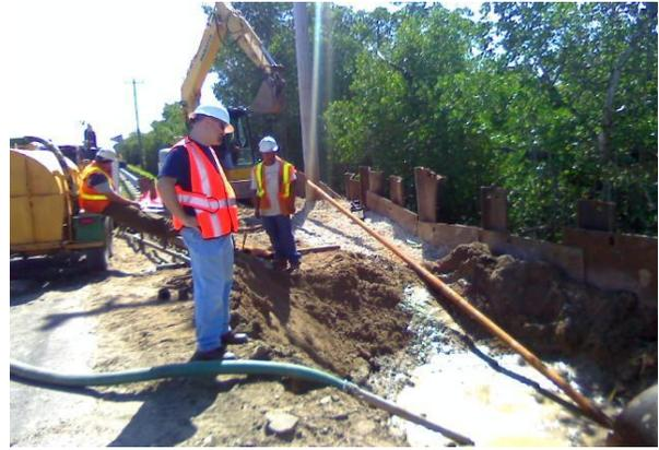
**Figure 3:** At the exit hole workers are placing a larger diameter reamer to widen the hole to fit the pipe.
