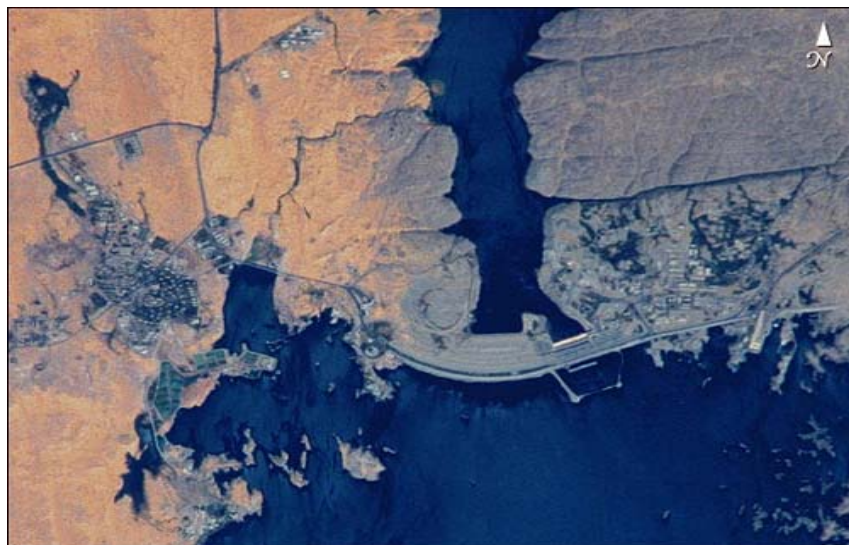
Figure 2.2 Aerial View of the Aswan High Dam
