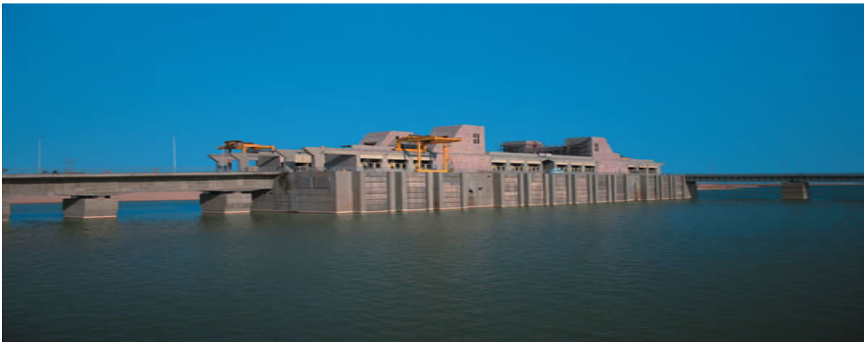
Figure 3.1 Digital Rendering of the Mubarak Pumping Station
