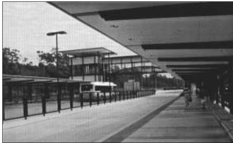
Figure 2. Griffith University Station, South Busway, Brisbane
