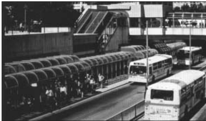
Figure 1. Tunney's Pasture Station, West Transitway, Ottawa
