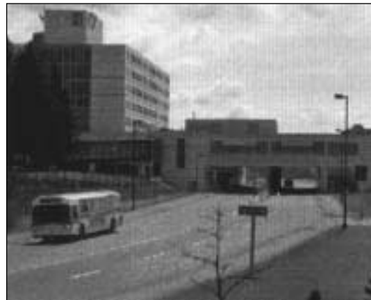
Figure 4. Riverside Hospital extends over a transitway station
