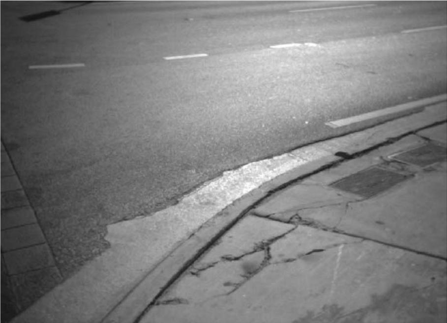
**Figure 9. Possible Damage on the Curb from Bus U-Turns**
